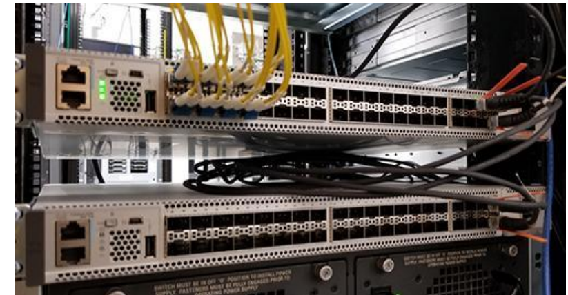
New core switch (located in MDF of High School)
